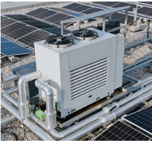
Rittal installed a chiller on the roof, ready to provide emergency cooling.
